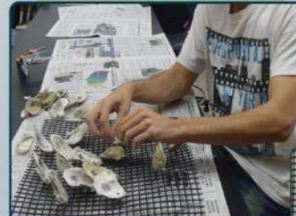
Volunteers drill holes in recycled oyster shell and attach them to mesh material in preparation for placement water-ward of the shoreline. These mats allow oysters to form reefs that protect the shoreline from erosion.
