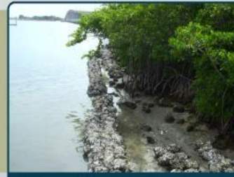
Oyster bags are stacked along the shoreline in front of these mangroves to create a natural buffer to waves, and protect the shoreline from erosion. The combination of oysters and mangroves (or other marsh plants) creates a living shoreline design.
