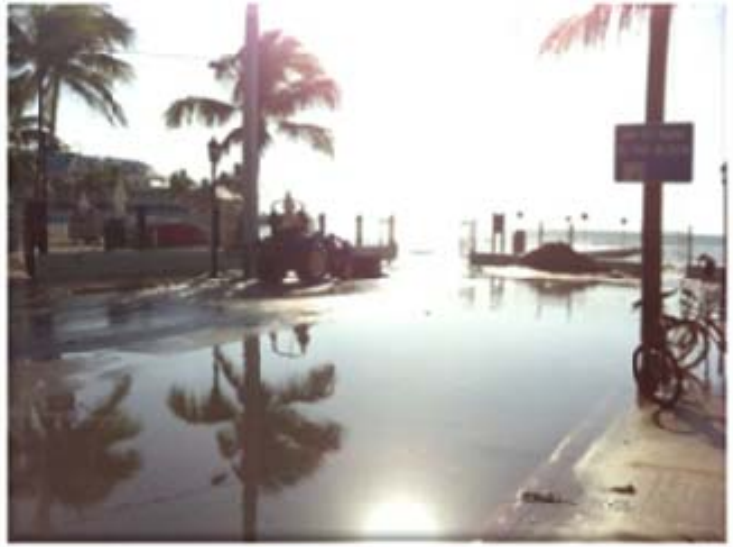
Duval Street high tide flooding
