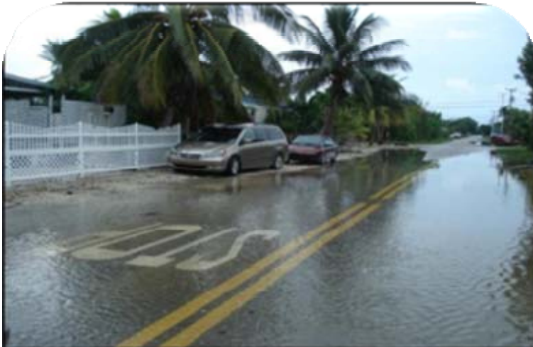
High-tide flooded road on Big Pine Key
