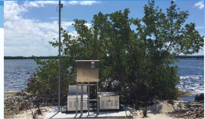
Before Hurricane Irma
