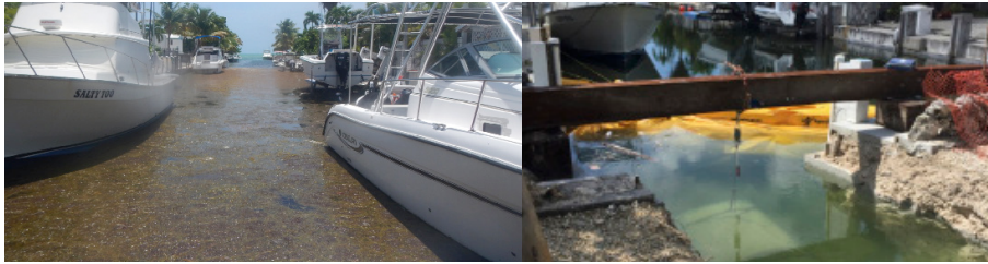
Left - Floating wrack in canal impairs water quality, Right - culvert dug to improve circulation, Page top - air curtain keeps out wrack
