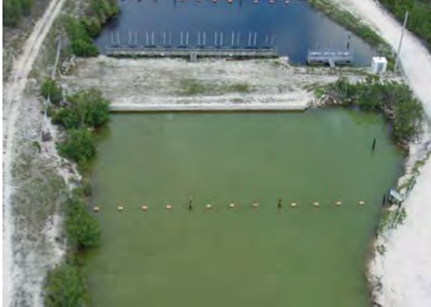
C-111 Canal discharge into Manatee Bay
