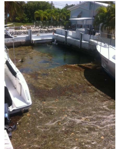
June 28 - culvert open
