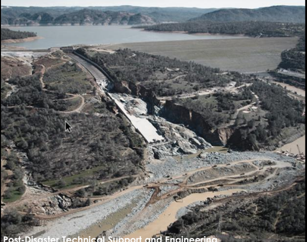
Post-Disaster Technical Support and Engineering Advice, Oroville Dam, California (FPMS)
